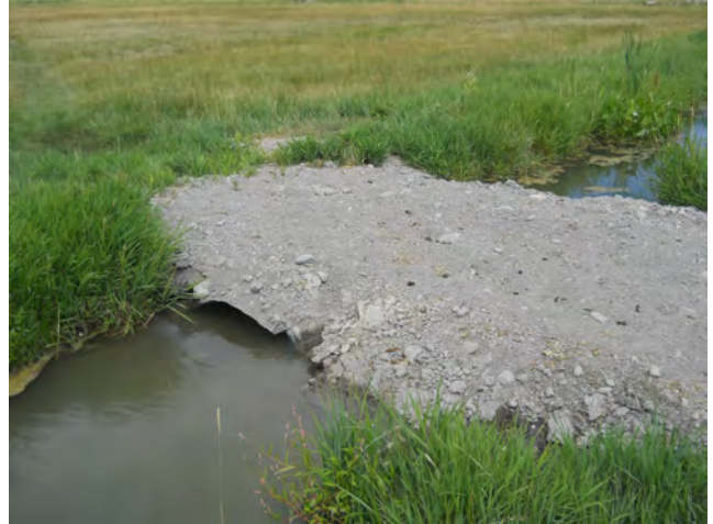
Figure 12. Site 42CA178, Feature 4, view to the northwest.
