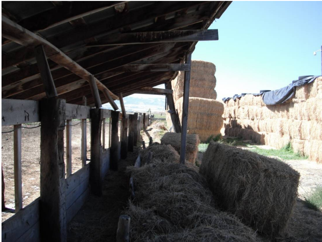
Looking at a covering over the animal feeding area and storage of hay bales adjacent to the northern animal corral near the north central portion of the subject property.
