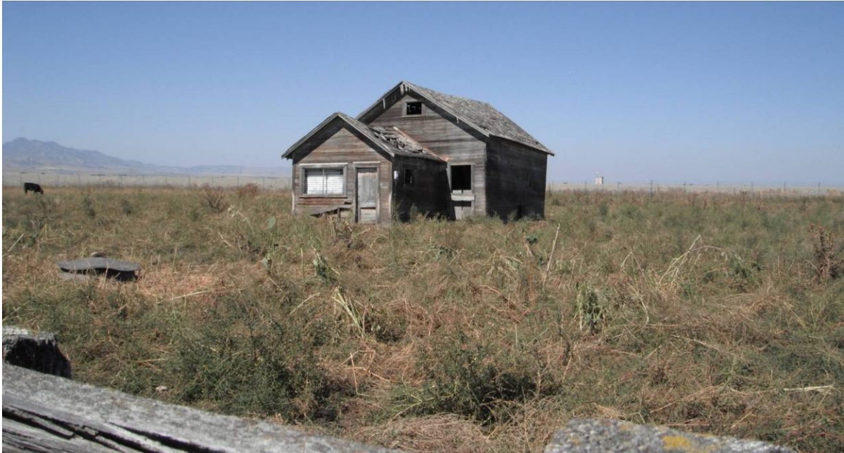
Looking north to northwest at an old, dilapidated, abandoned wooden home on the subject property near the central portion of the northern boundary of the subject property.
