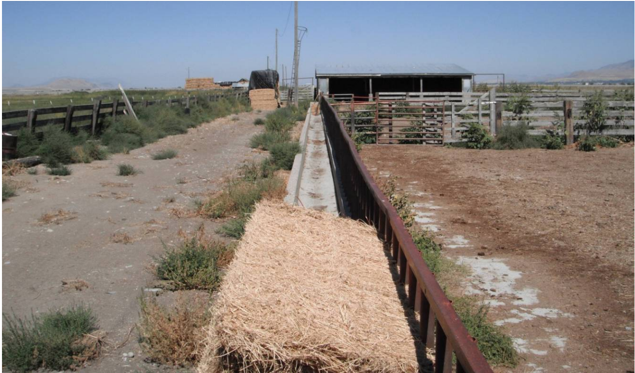
Looking north along the western portion of the southern animal corral located in the south central portion of the subject property.
